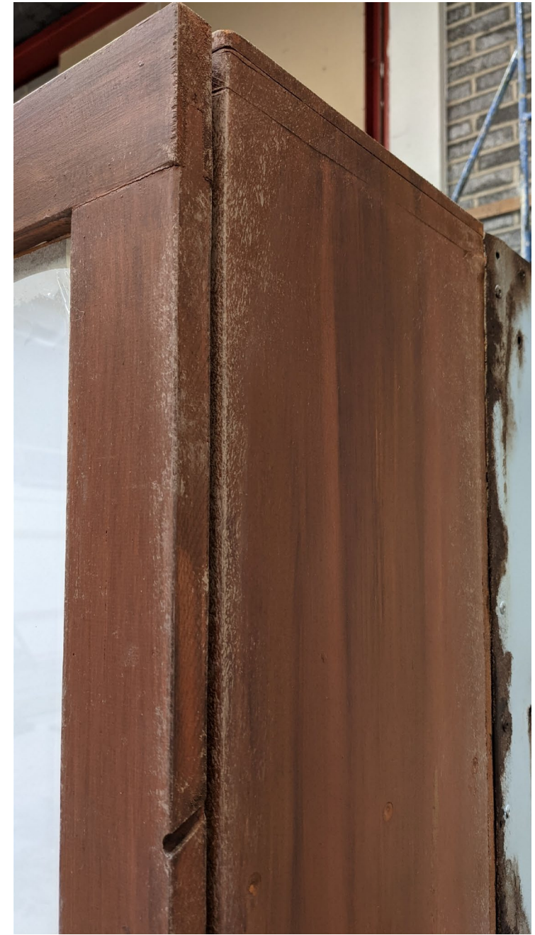
Creating a wood grain effect for the shelves and benches using washes and glaze, with rollers to age and finish.
